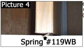
6. Attach the acoustic seal Spring #119WB on the bottom rail of the door. (Picture 4 and technical drawing)
