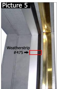
Now install the acoustic seals on the two jambs. Then attach the **Snap-On Covers** (technical drawing) **before installing the acoustic seal on the head**.
