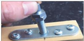
**10.** Raise the door and screw the roller bolt into the mounting plate on the top of the sliding door. →
