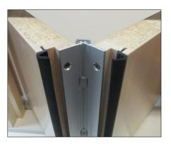
7. Center a mounting plate on the top of the pivoting door with the flat side facing out. Using the starter holes, screw it in place ♥ with 32-mm (1-1/4-in.) no. 10 screws.
